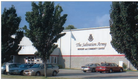
Figure 34-5 The Salvation Army is a voluntary agency that provides full-scale community services.
